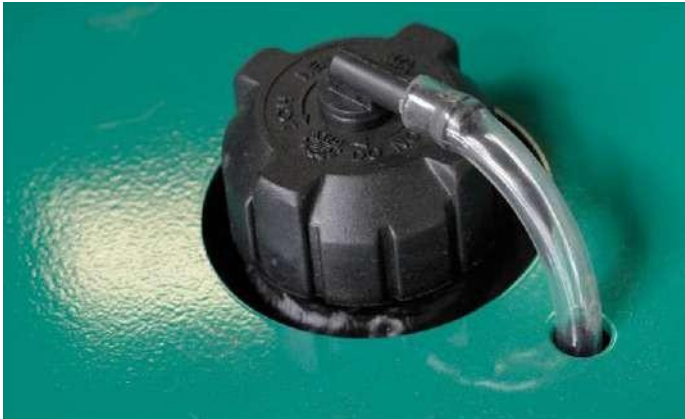
Figuur 6.4 | koelwater vul opening
